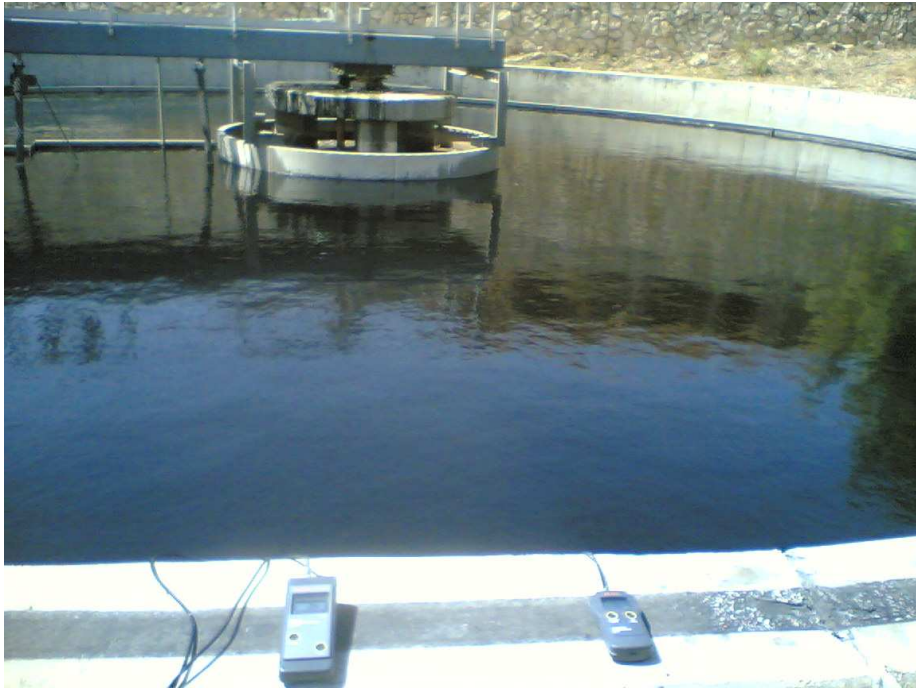
Figure 61. The Sedimentation tank (1) in the summer (July, 2010)
