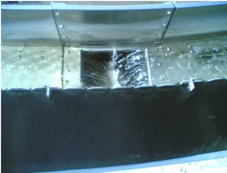
Figure 62. The effluent from the sedimentation tank (2) (June, 2010)
