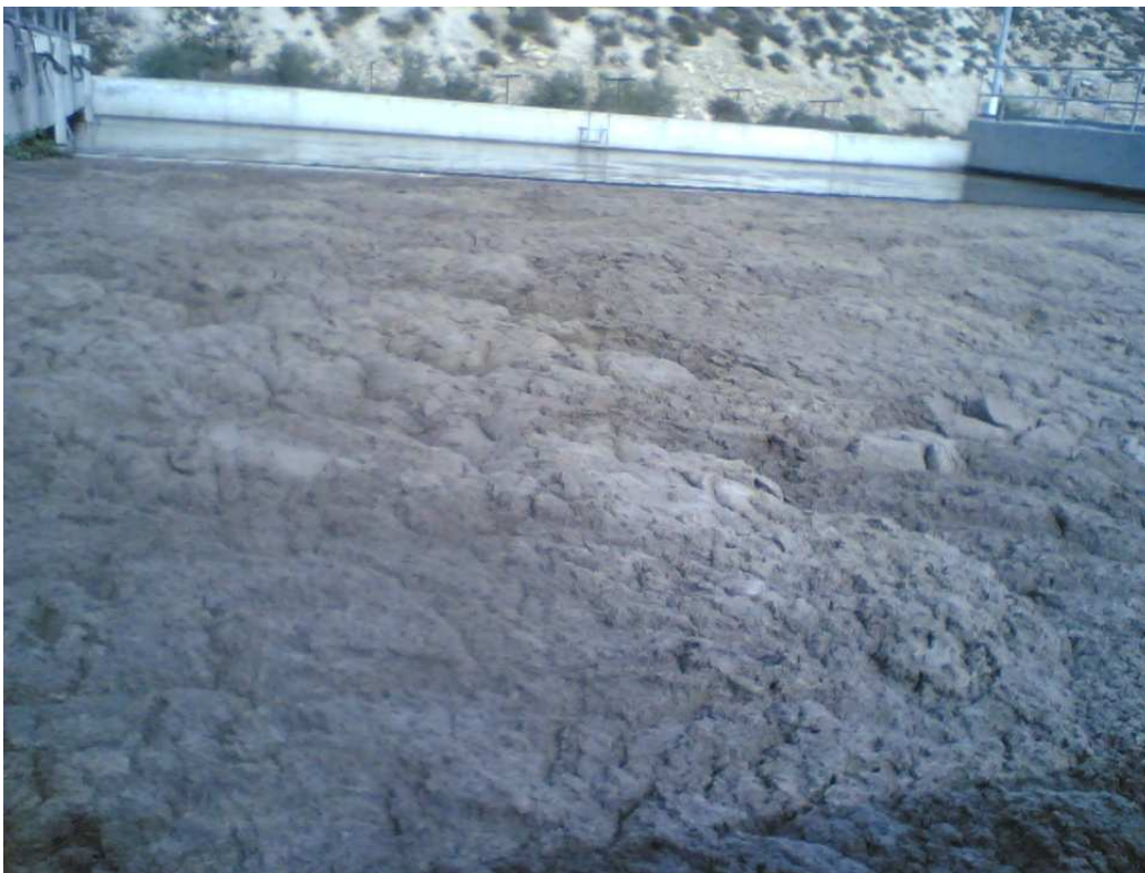
Figure 1. The foam in aeration tank (2) in AWWTP (March, 2010).
